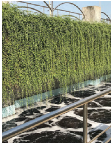
Bio-organisms eat suspended and dissolved solids from the dye as it passes through the system.
